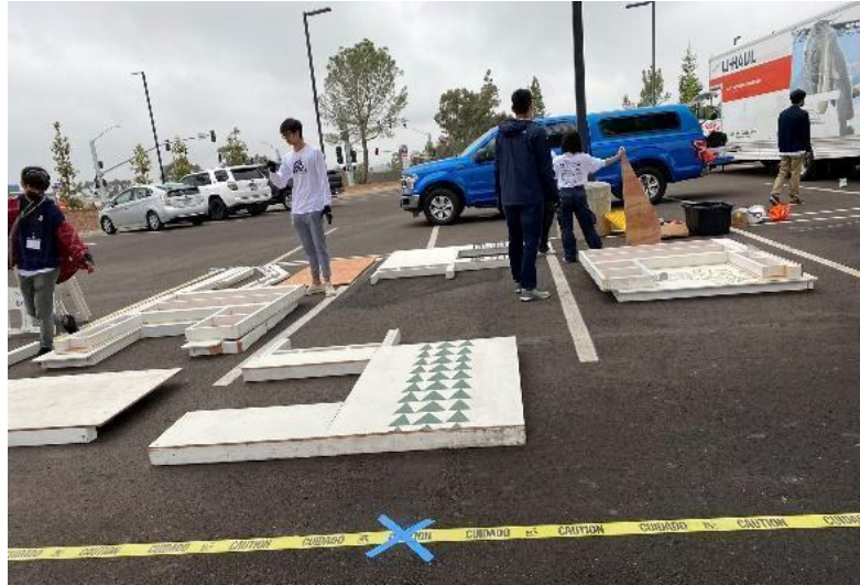
Example of panelized walls at 2022 TSDB
